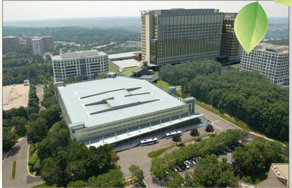
Artist's drawing of the completed facility showing the East Tower, the West Tower, South Parking Garage, North Parking Garage, the Transportation Center, and the Remote Inspection Facility. (Photo by Marc J. Barnes)
